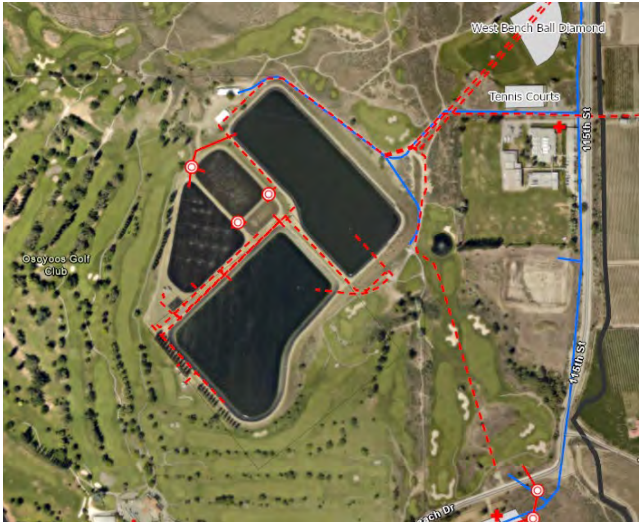
FIGURE 1-1: OSOYOOS AERATED LAGOONS AND RECLAIMED WATER STORAGE
