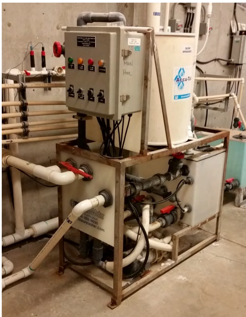
FIGURE 6-2: CALCIUM HYPOCHLORITE MAKE-UP AND DOSING SYSTEM
