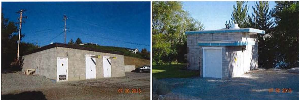
FIGURE 3-2: IRRIGATION SYSTEM PUMPHOUSES, INTAKE #9 (LEFT) AND INTAKE #8 (RIGHT)
