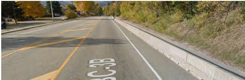
Figure 3-13 Highway 3B, Trail BC Source: Google Street View Image Capture 2018 (2022)
