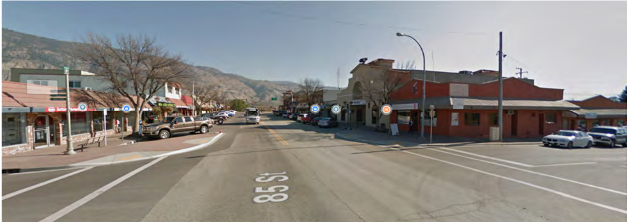
Figure 2-6 Existing Pedestrian Sidewalk on Main Street Eastbound at 85 Street. Source: Google Street View Image Capture 2018 (2022).
