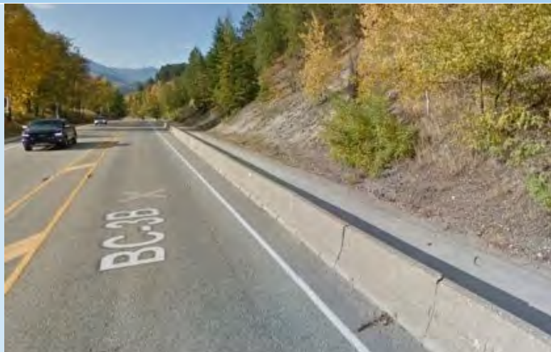
Example of paved shoulders along Highway 3 in Trail
