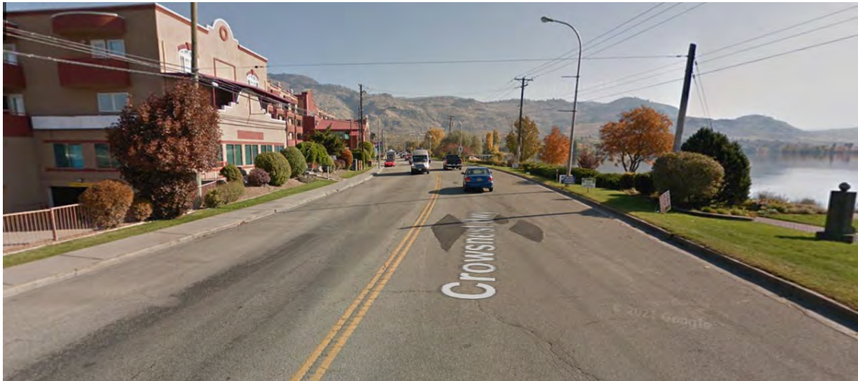
Figure 3-9 Existing Cross-Section Main Street/Highway 3 Eastbound. Source: Google Street View Image Capture 2018 (2022)
