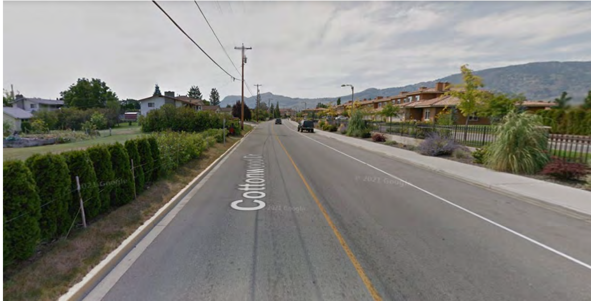
Figure 3-11 Existing Cross-section Cottonwood Drive. Source: Google Street View Image Capture 2012 (2022)
